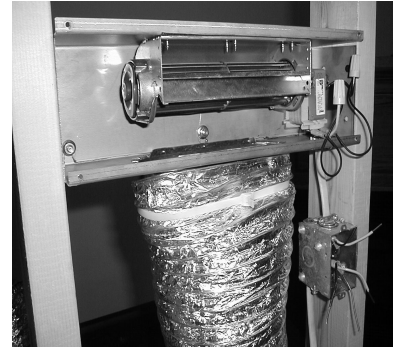
Figure 9.6, Secured Duct Pipe
